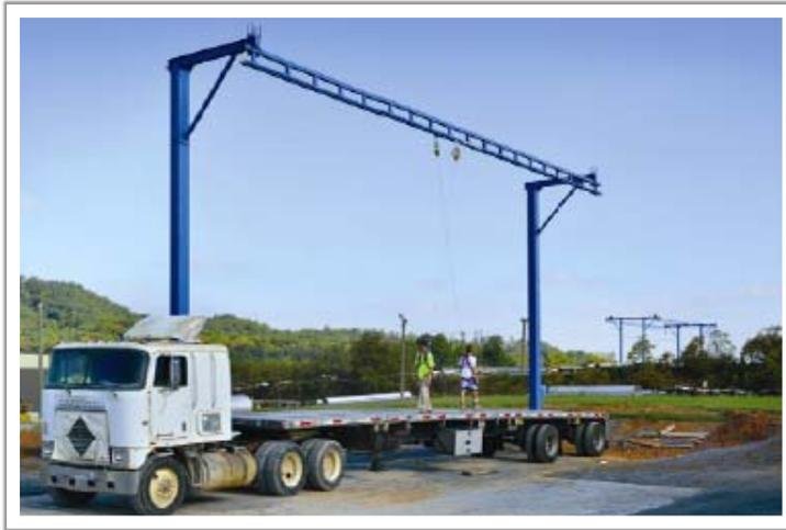
They found a solution, with a lower cost than a new building and allowed the workers to remain on the truck, in the form of two free standing Tether Track fall protection systems by Gorbelt. The primary system features two cantilevered monorails, which enables two flatbeds to be loaded in the same area simultaneously. Each monorail uses Gorbelt's dual track, allowing two workers to pass one another safely without disconnecting the lanyard from their harness. A second Tether Track system
