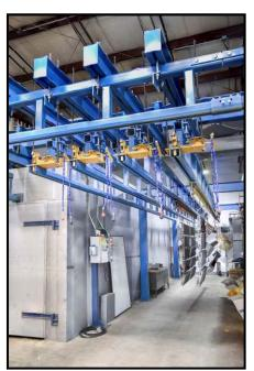
Knowing the high quality of the Gorbel® product lines firsthand, they chose a Gorbel® Freestanding Work Station Crane to maximize throughput while providing a safer and more ergonomic process for their paint department. The structure has a 4000 pound capacity with 2000 pound bridges and monorails. The two bridges each are twenty-seven feet eight and one quarter inches in length. The runway length is forty-seven feet, ten inches.
