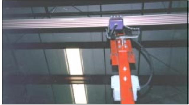
Four-Bar replaced the festoon systems on four transfer car runways in this plant, as well as additional runs in a second plant. Owners are happy with the trouble-free performance of the Four-Bar.
