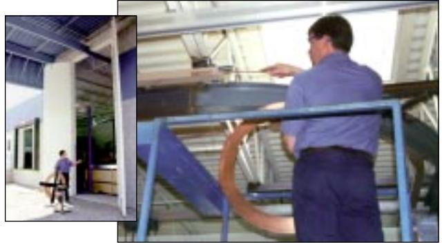
The Tri-Bar and Four-Bar conductors are supplied in coils, and inserted in the housing slots from one end of the run. Long runs are coiled on a cross for added stability and to use with payoff stands.
