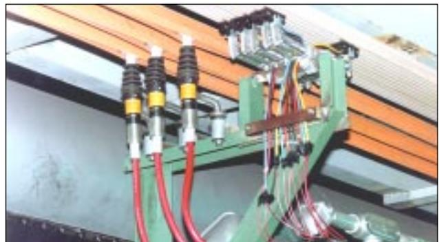
10 control lines require less than 7 inches of space for this steel slab grinder, using Tri-Bar and Four-Bar. Universal's Span-Guard, shown, provide the main power.
