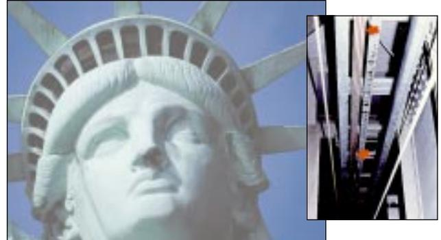
The service elevator on the Statue of Liberty uses a vertical run of Four-Bar for power. Important features are reliability and compactness for this 245 foot high run.
