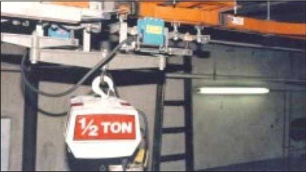
This monorail system shows a Tri-Bar entrance guide and a Power Pickup on a disengageable base. The hoist is entering an electrified zone for a hoisting area.
