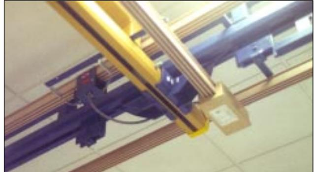
The Power Pickup on this light duty crane runway feeds power to the bridge track. The drag on the manually pulled hoist is negligible.
