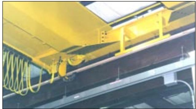
The Four-Bar provides continuous copper bars, joint-free for the entire runway length. Four conductors take up only 2 5/8 inch of horizontal space.
