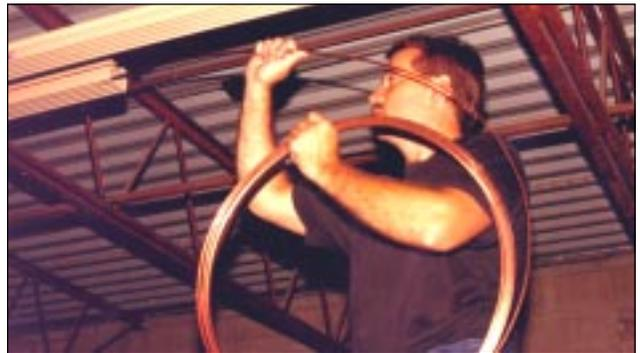
The key to superior performance is eliminating joints in the conductors. The copper conductors come in coils, as shown, and are slid into the housing from one end of the conductor system.
